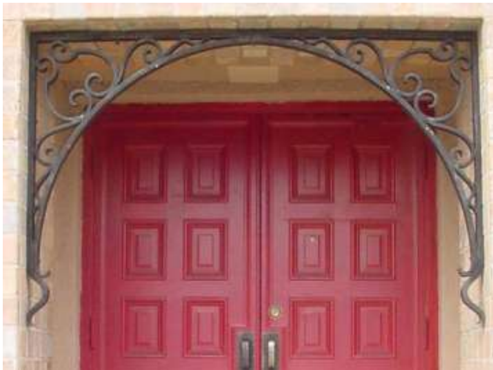
Left: Wrought iron insert brackets at Main Parish Hall entry.
