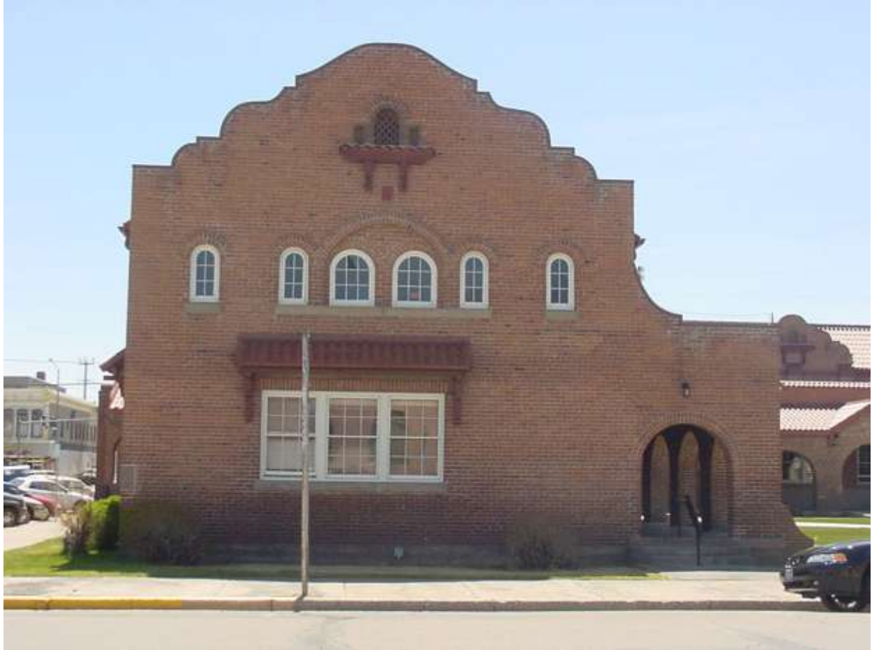
Alamosa County Courthouse, with Mission Style inspired parapet detail.
