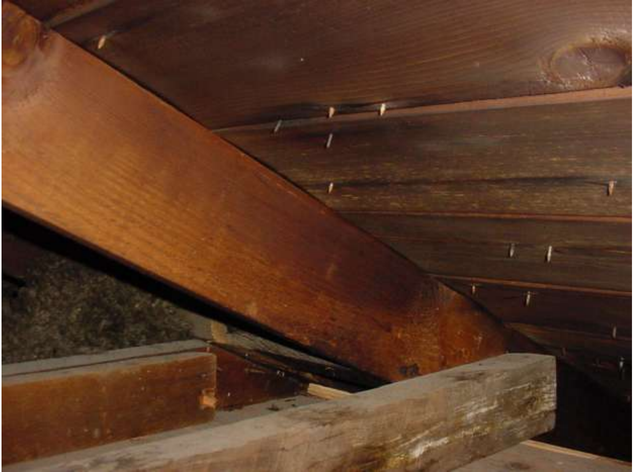
Sanctuary attic condition, showing field assembled truss.
