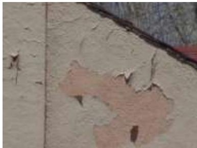
Peeling paint over stucco..
