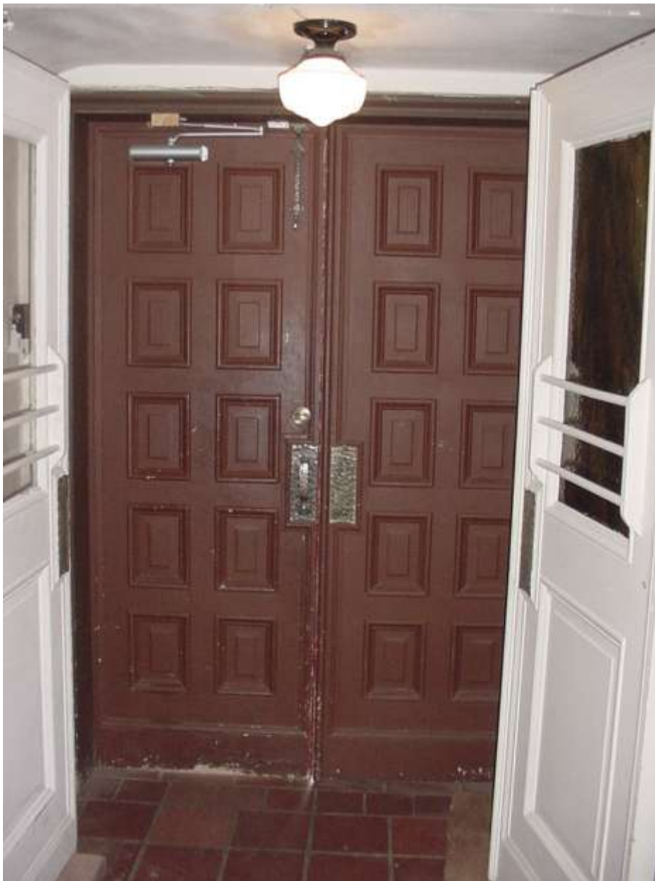
Parish Hall entry doors at interior.
