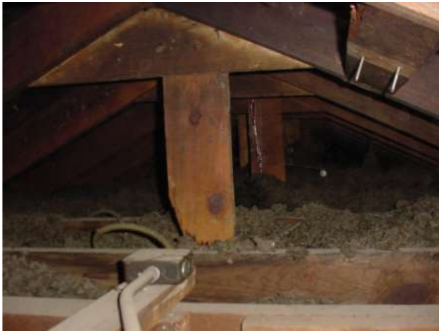
Sanctuary 2x6 field-assembled trusses, with various wood bridging and truss plates.
