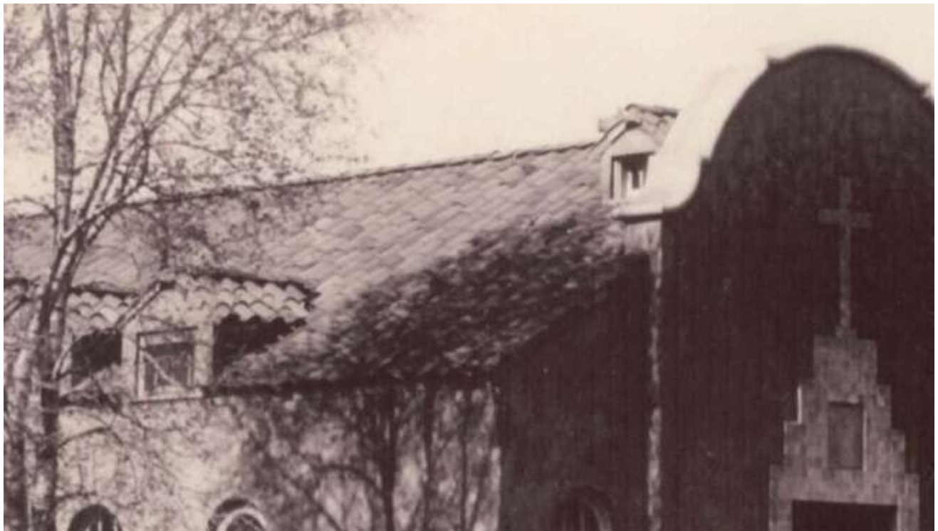
Detail at original clay tile roof.
