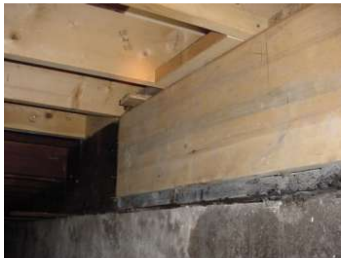
Floor framing at chancel.
