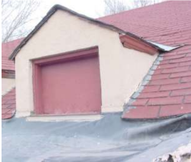
Sealed dormer at west side of Parish Hall. Dormer at east side of Parish Hall.
