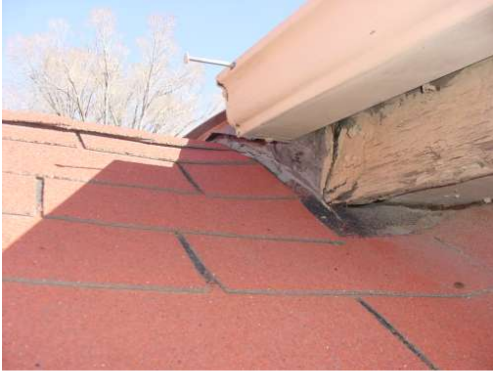
Wood trim at wall/ roof intersection at side Sanctuary entry.
