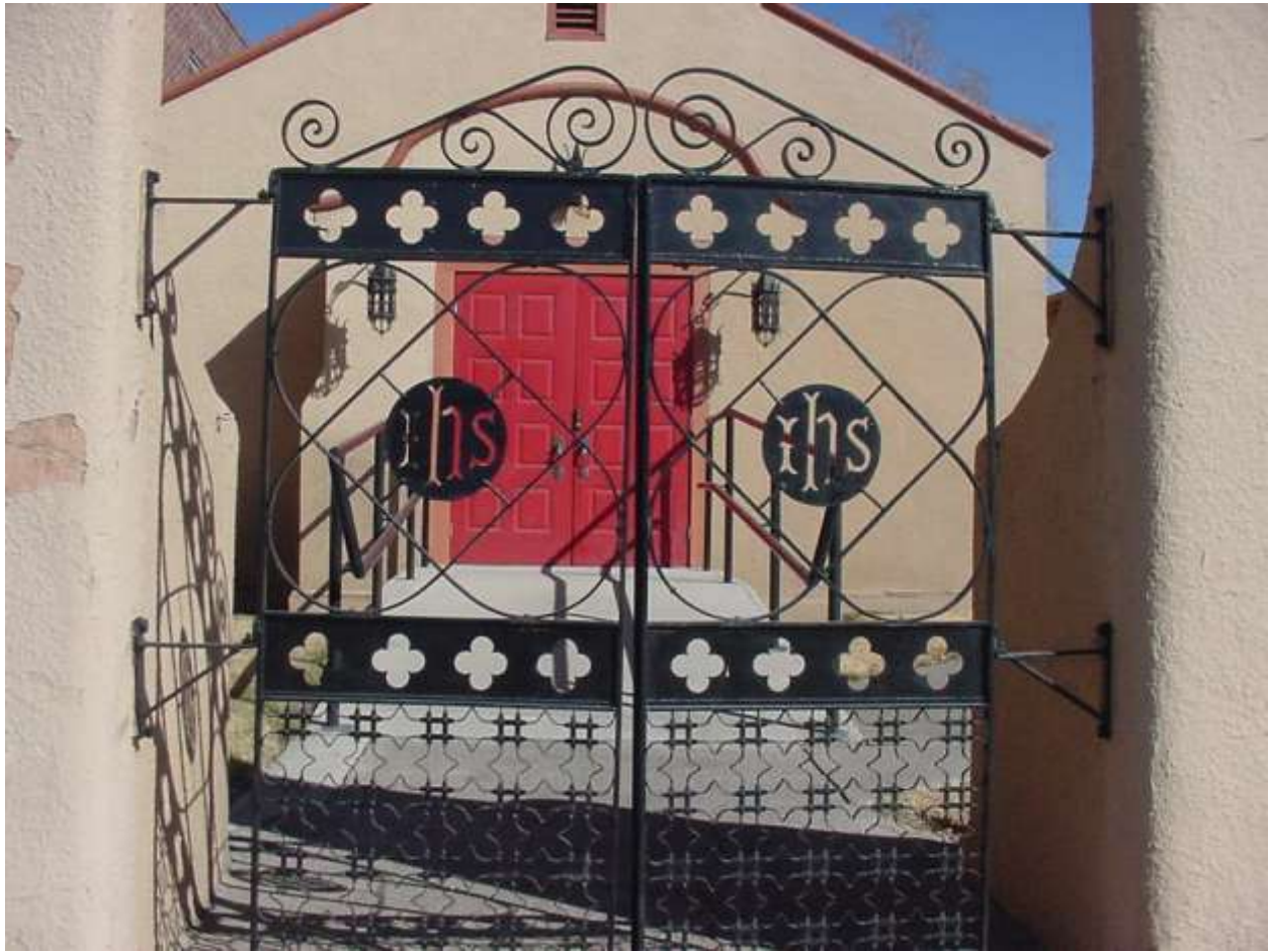
Iron gate at Sanctuary main entry.
