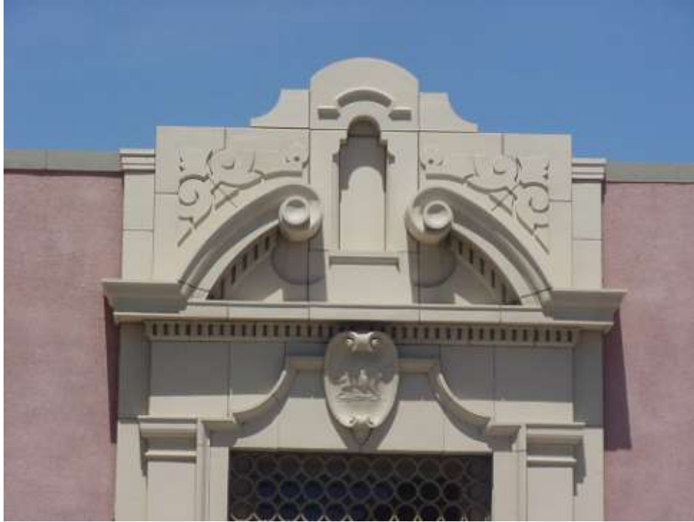
Eclectic frontispiece and parapet detailing at former Alamosa Post Office.
