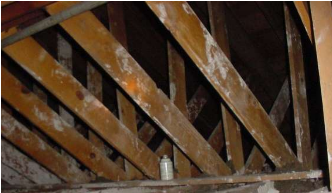
Roof trusses at Parish Hall.
